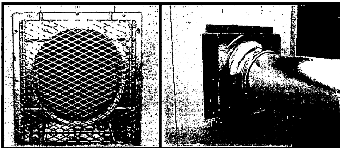
Figure 2 - Exhaust Duct to Capture Emissions from the Process.
